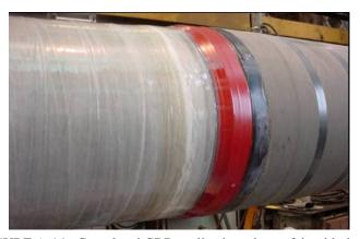
FIGURE A-14. Completed GRP application, shown fair with the sleeve.
