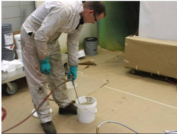
FIGURE A-4. Pre-mix of the elastomeric coating components.
